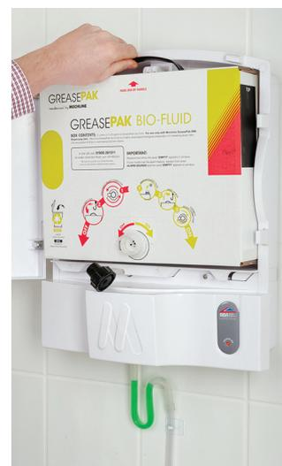
*why fix it?"* With the Mark 1 model staff are notified that the fluid needs replacing by a red 'empty' notification on the front of the unit, whereas in the later Mark 2 model an audible alarm alerts operators to the fact it needs changing. Both features prompt timely and efficient maintenance, so operators don't have to remember.
