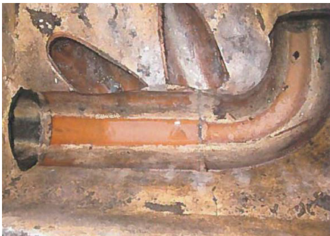
The clear sewer run at the end of the year-long trial, April 2017.
